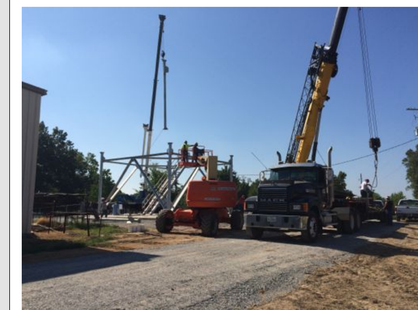
65-ft tower construction began Sept. 1, 2015
