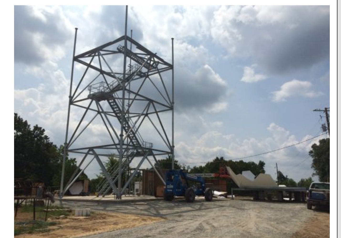
Tower complete and radome construction began Sept. 11, 2015
